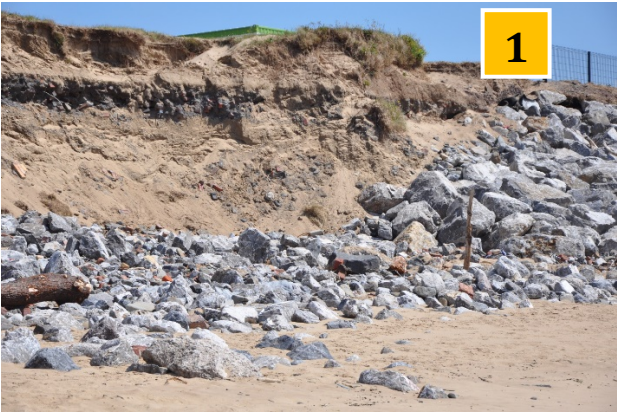
Figure 2 - Pedestrian access to the beach at West end of weldmesh fence
